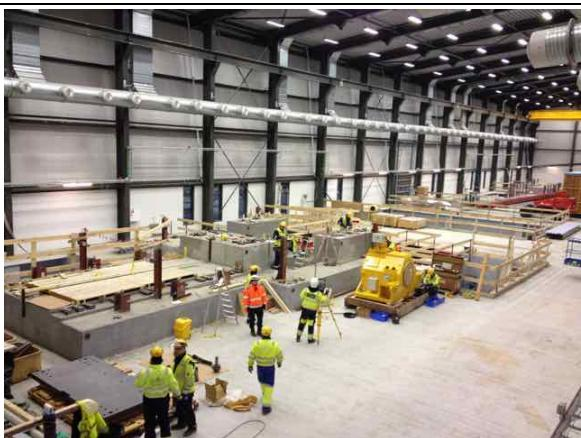
Photo 73: Turbine and generator platforms under preparation
