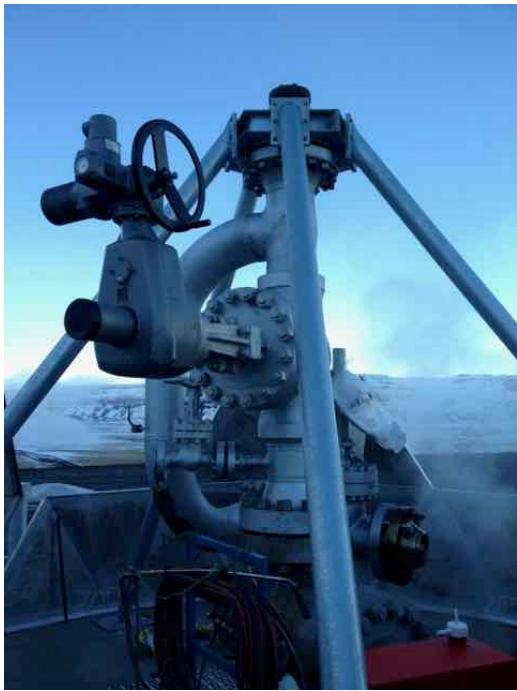
Photo 48: Wellhead valves
