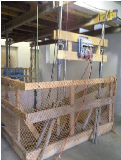
Photo 82: Temporary protection of stairwell
