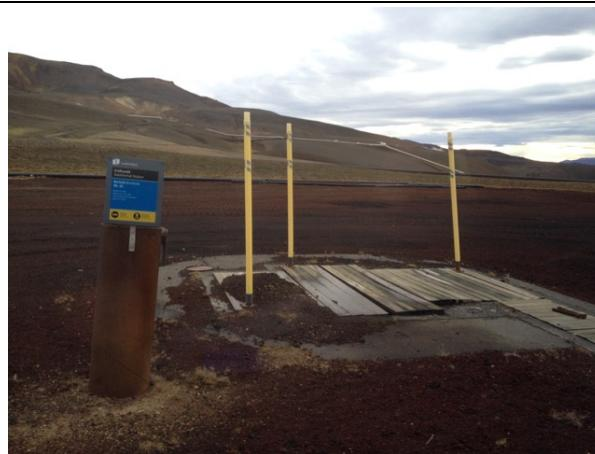
Photo 86: Closed wellhead from deep drilling project at Krafla
