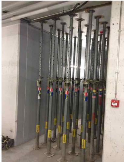
Photo 80: Supports in basement for heavy turbine transport above
