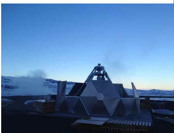
Photo 47: Wellhead protection dome under assembly
